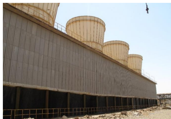
Fig. 2. General view of the studied cooling tower.
