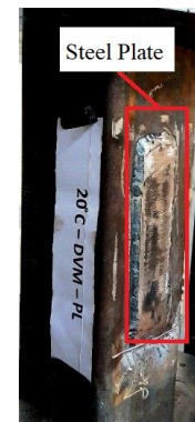
Figure 1. Retrofitting of column specimens by steel plate
