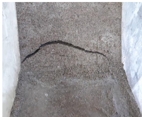
Fig. 3. Failure shape with 5% nano-lime covering
