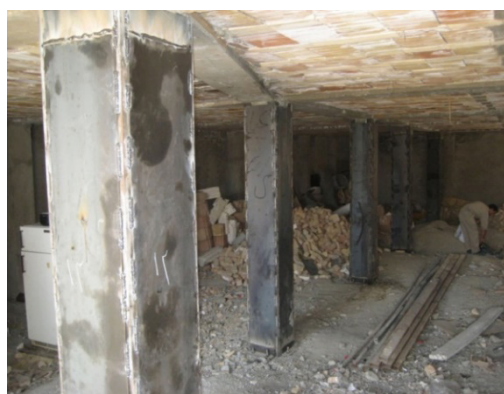
Figure 5. Steel jacket retrofit of square RC columns
