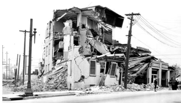
Fig. 1. URM collapse, Long Beach, California 1933 [1]
