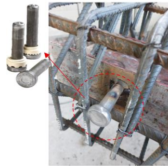
Figure 1. Details of Shear Studs
