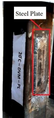
Fig. 1. Retrofitting of column specimens by steel plate
