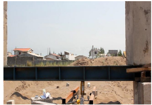
Fig.1. A view of pile load test
