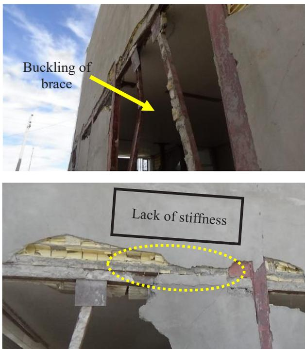
**Fig. 2. (Top) buckling of brace in out-of-plane, (Bottom) lack of stiffness in link beam (Authors)**
