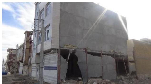
Fig. 1. Damaged three-story building with EBF system in the Sarpol-e Zahab earthquake (Authors)
