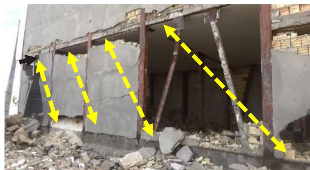
**Fig. 3. Tolerate part of the lateral load by the formation of the compression diagonal struts of infill walls (Authors)**
